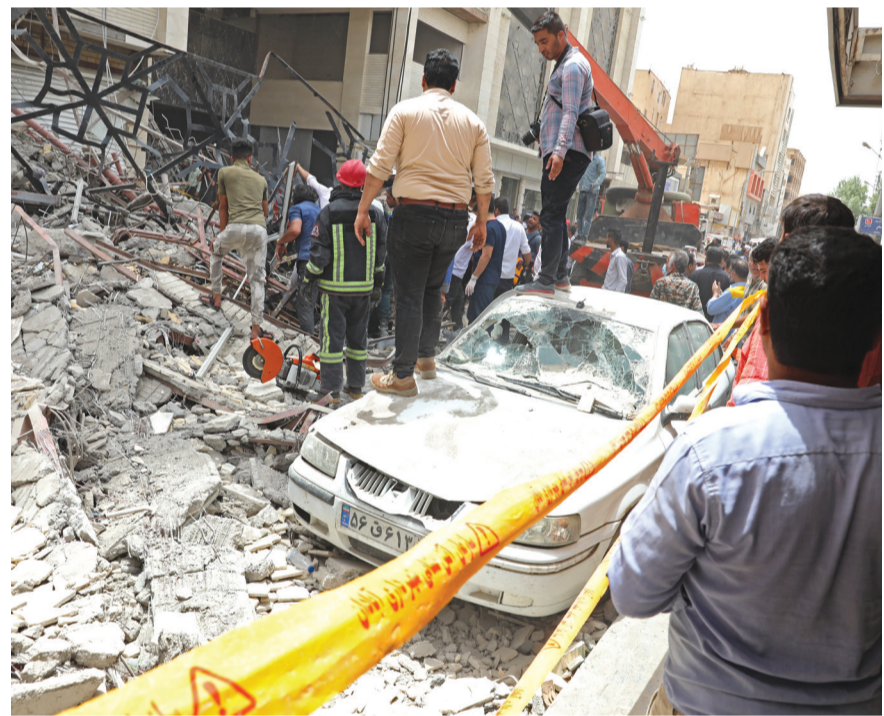
Iranians gather at the site where a ten-story building collapsed in the southwestern city of Abadan on May 23, 2022. At least four people died and about 80 were trapped under rubble when an unfinished building collapsed in southwestern Iran, officials said. (Photo: AFP)
